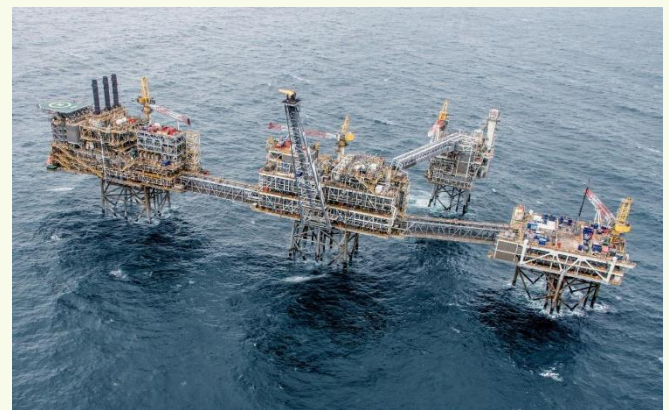
Figure 5 – Buzzard Production Platform in the North Sea
