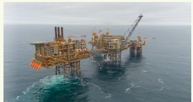
Figure 4 – Golden Eagle Production Platform in the North Sea
