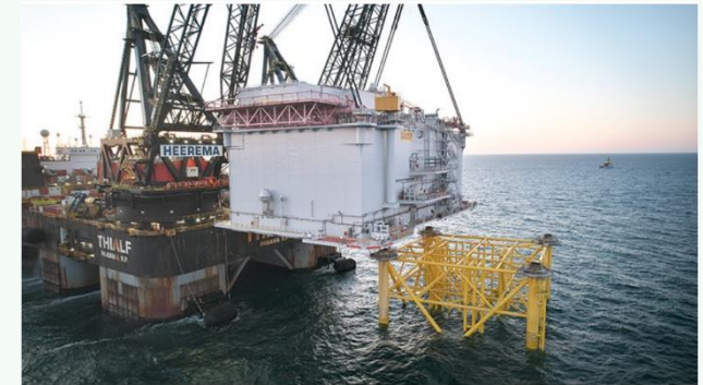
Figure 57 - HVDC substations being installed at Dogger Bank (SSE Renewables, 2023)
